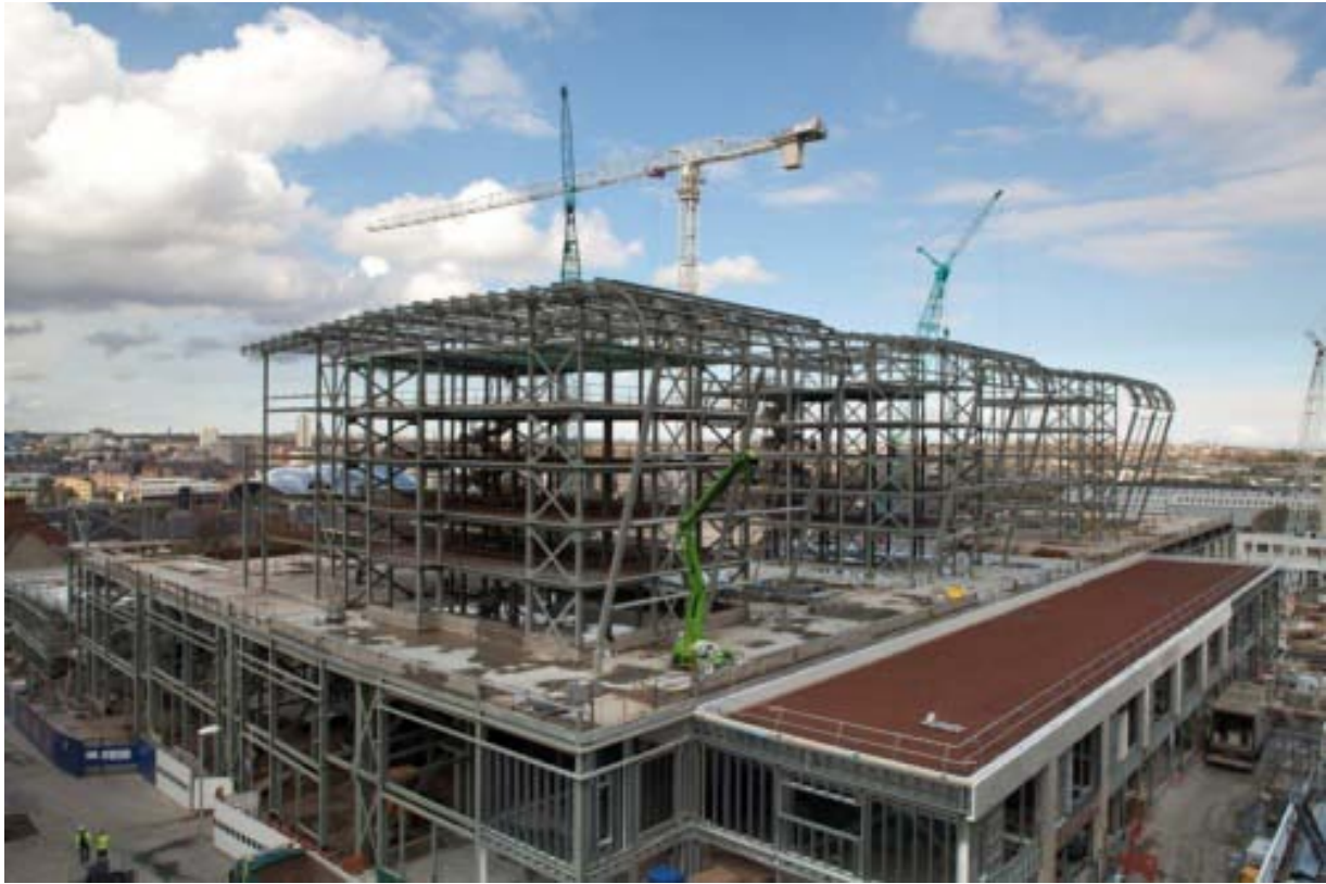
Fig 5 – Erection Assembly (3-Erect-Asmb)
